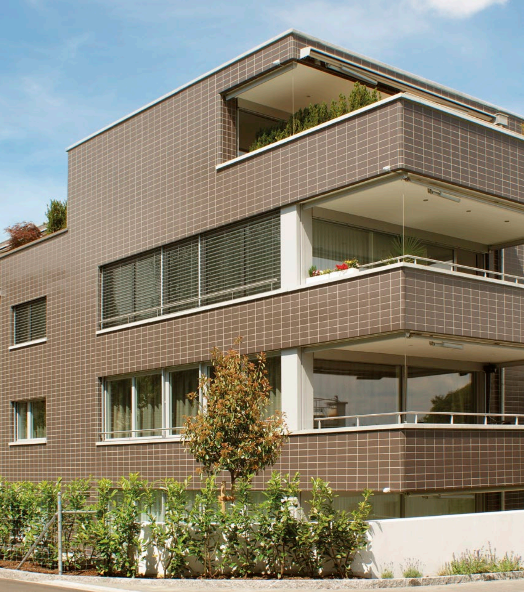
Apartment building, Kilchberg, Switzerland / Horizon Architektur + Bau AG, Zürich, Switzerland
