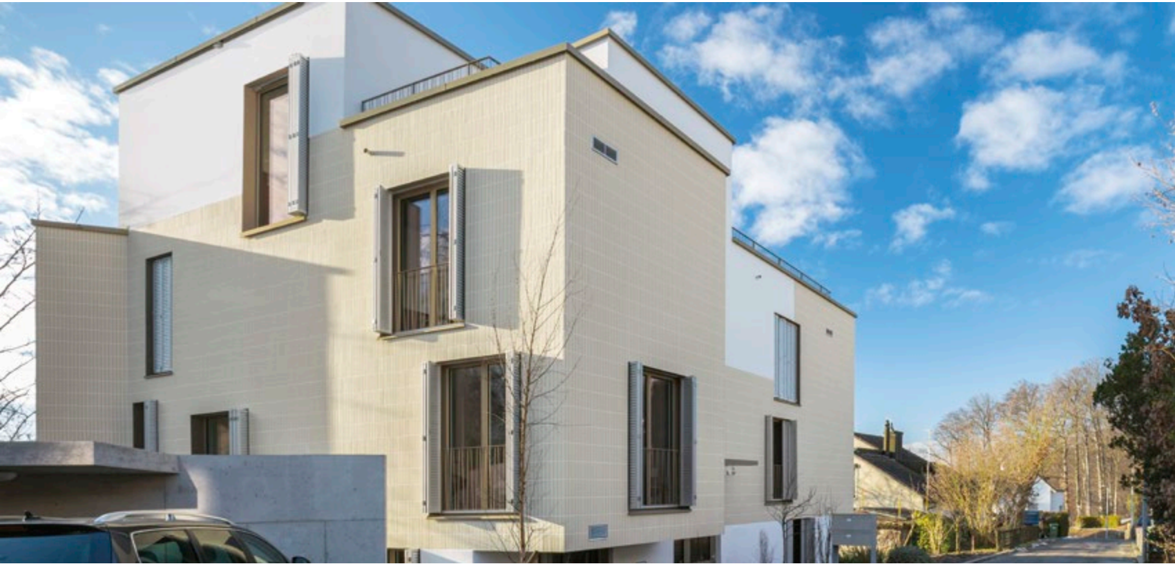
Apartment building, Zurich, Switzerland / Kissling + Roth Architektur, Zurich, Switzerland
