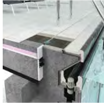
Large overflow channel with handhold-piece.
