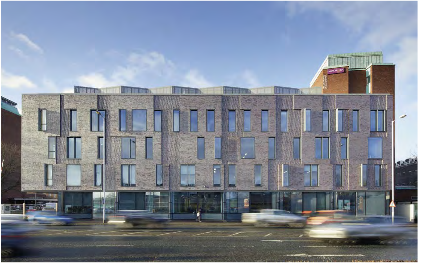
SCHUSTER ANNEXE, UNIVERSITY OF MANCHESTER, GB HAWKINS\BROWN ARCHITECTS, MANCHESTER
