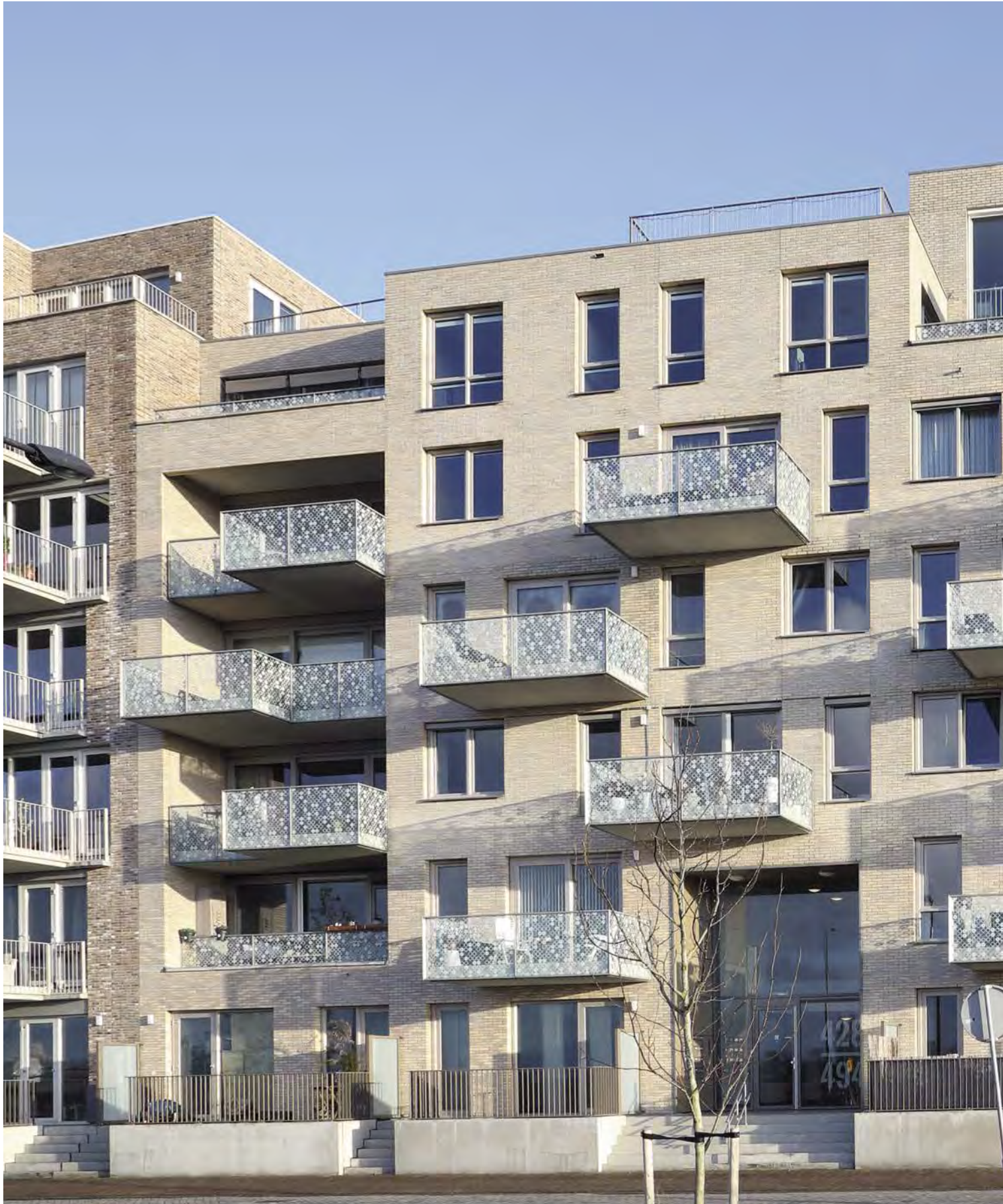
Y-CITY BLOCK 15, AMSTERDAM, NL JUST ARCHITECTEN TE AMSTELVEEN
