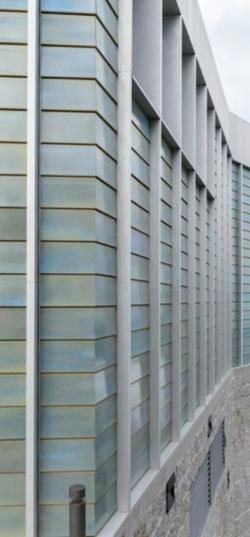
Meanwhile, back at **City Village** the tallest of the four volumes on the scheme that rises above the city – a 20-storey tower – is at once designed to stand out and disappear by being designed with the same cladding composition as the other terracotta elements, but carried out in a high-gloss light blue terracotta tile. The tower reflects the colors of the cityscape and sky, giving the project an unexpected lightness. Photos: Simon Hadley
