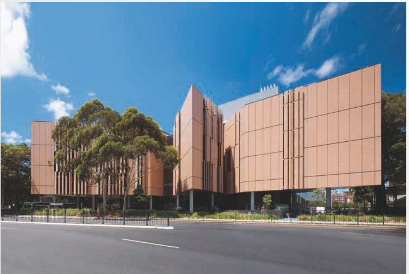
tempio®[projects] UNSW University of New South Wales Sydney, Tyree Energy Technologies Building. Sydney, Australia.
